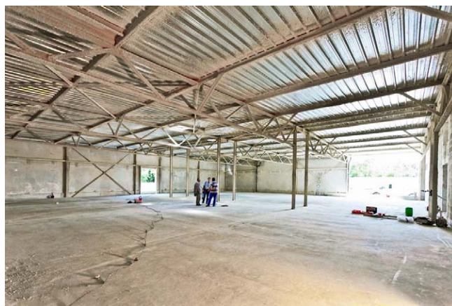
Located in the secure Locarchives records storage complex, the new Corbis/Sygma facility will have three separated humidity-controlled cold storage vaults, with a total storage area of 500 m 2 .
