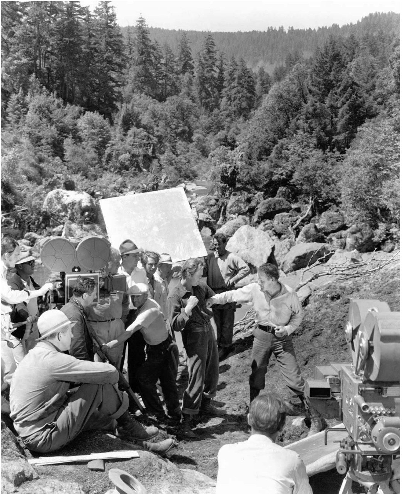
Technicolor three-strip cameras on location in Eureka, California filming the Warner Bros. 1938 feature Valley of the Giants . The wide film magazines on the cameras carried three rolls of black-and-white separation negative film. Brilliant color prints were made from the negatives by the dye-imbibition (dye transfer) process in Technicolor's laboratories.
