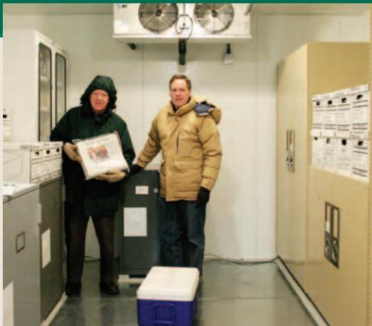
*Henry Wilhelm (left) and Mark McCormick-Goodhart in Wilhelm Imaging Research's sub-zero cold storage vault, designed to preserve archival materials. The vault's "Sealed-Cabinet" cold storage technology (developed under a three-year project funded by the Smithsonian) eliminates the need for expensive, maintenance-intensive dry desiccant dehumidifiers to control relative humidity, and greatly reduces the costs of construction and electricity.*
