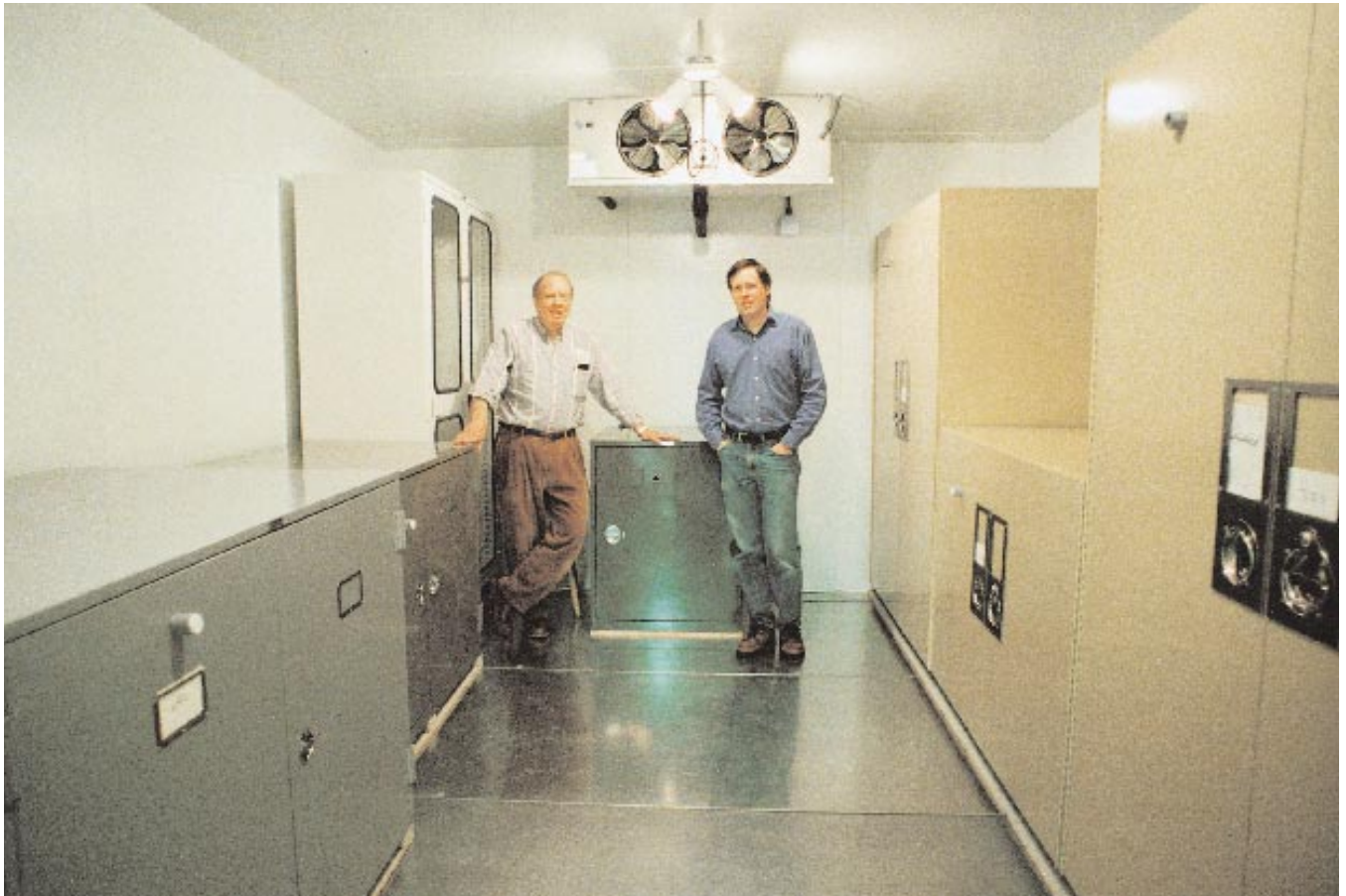
Henry Wilhelm (left) and Mark McCormick-Goodhart stand in the cold storage vault at Wilhelm Imaging Research Inc., in Grinnell, Iowa. The vault is part of a three-year research project in preservation for the Smithsonian Institution in Washington, D.C. The doors of the cabinets that line the walls are fitted with sealing gaskets that protect the negatives, film, and prints stored within the freezer units.
